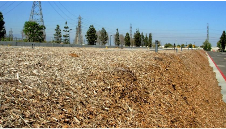
Proper operation of the facility, including maintenance of the biofilter, is often the key to reducing odor generation and movement offsite.
