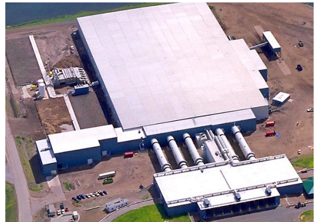
Facility design must take into consideration odor management and the quality and marketability of the finished product. Photos courtesy Ron Alexander
